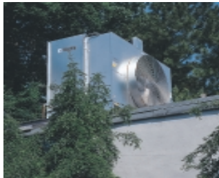
Figure 36: Fluid cooler cross flow with self-contained sump.
